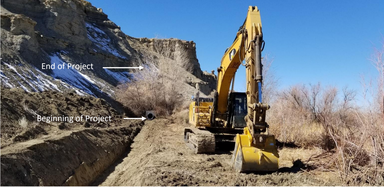
Project Site (Beginning of Project Looking West)
