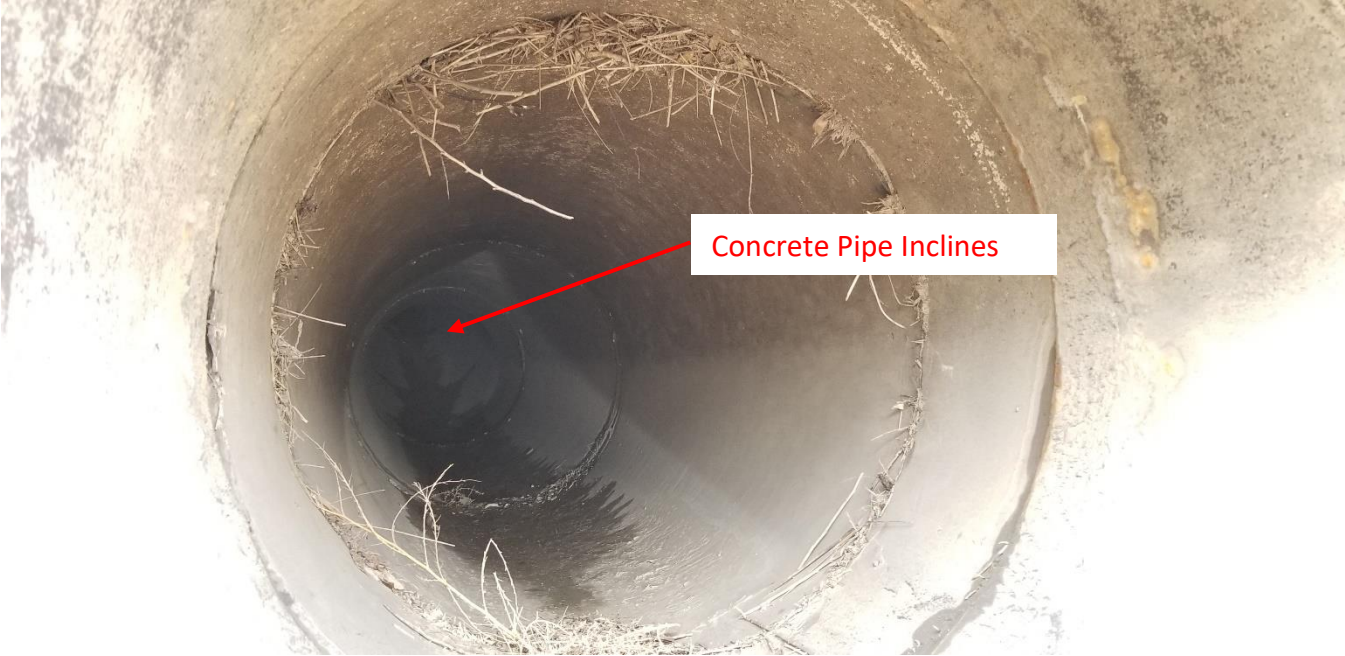
Project Site (Beginning of Project Looking into 36-inch Concrete Pipe)
