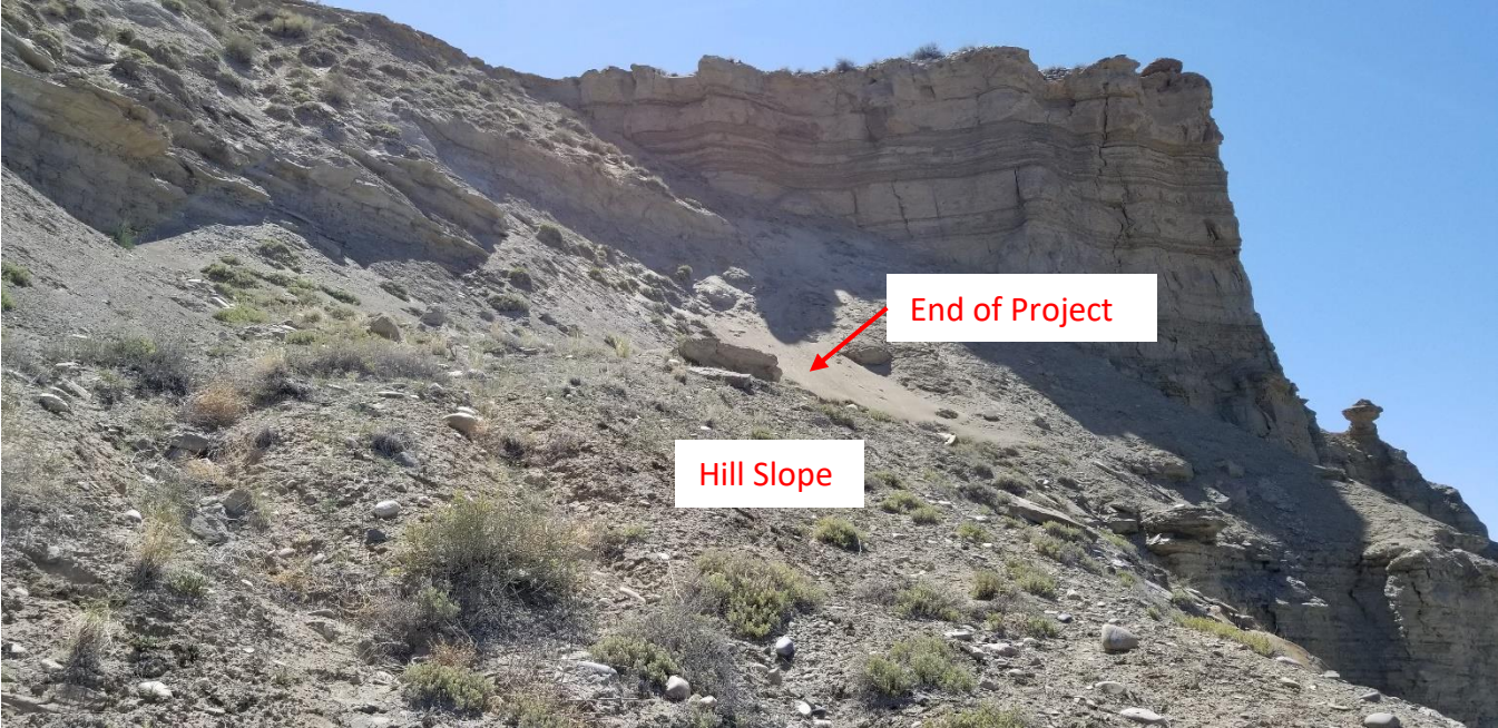
Project Site (Looking West Uphill Towards End of Project)
